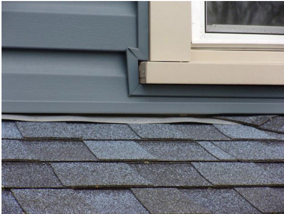
Roofing: Flashing at low roof
