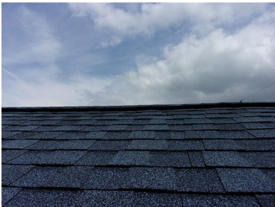
Roofing: Ridge vent installed
