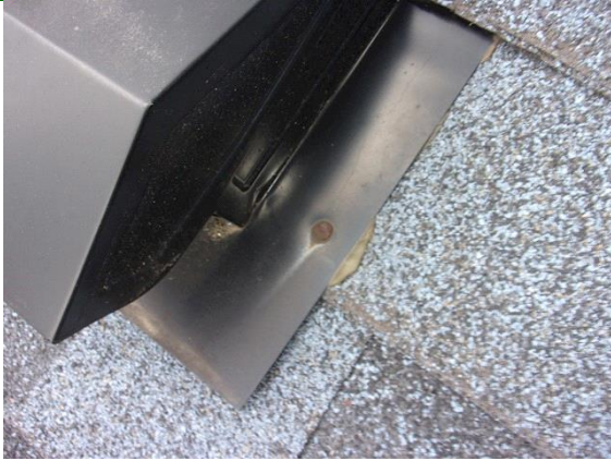
Roofing: Bath vent flange nailed and sealed
